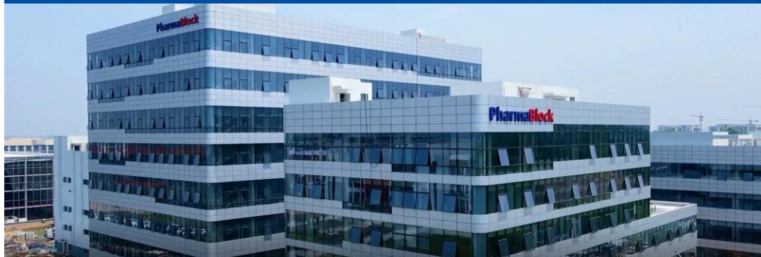
New CDMO Process R&D Center, 679,000 ft 2 \ 1000+ hoods
