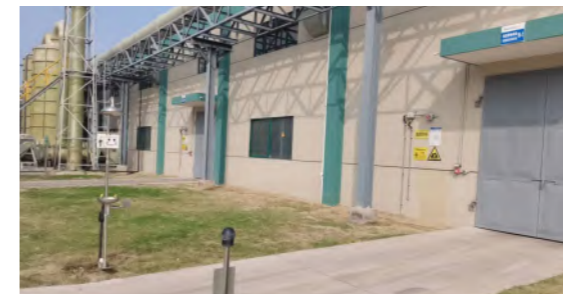
Hazardous solid waste warehouse
